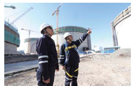
□ Receiving Terminal Phase-II Project of Tangshan LNG Project
