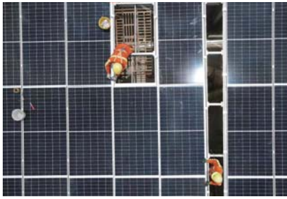
□ Photovoltaic field construction
