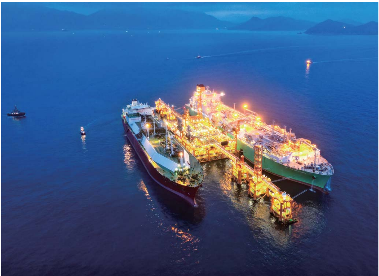
□ Project completion and delivery of Hong Kong LNG Receiving Terminal, the world's largest offshore LNG receiving station
