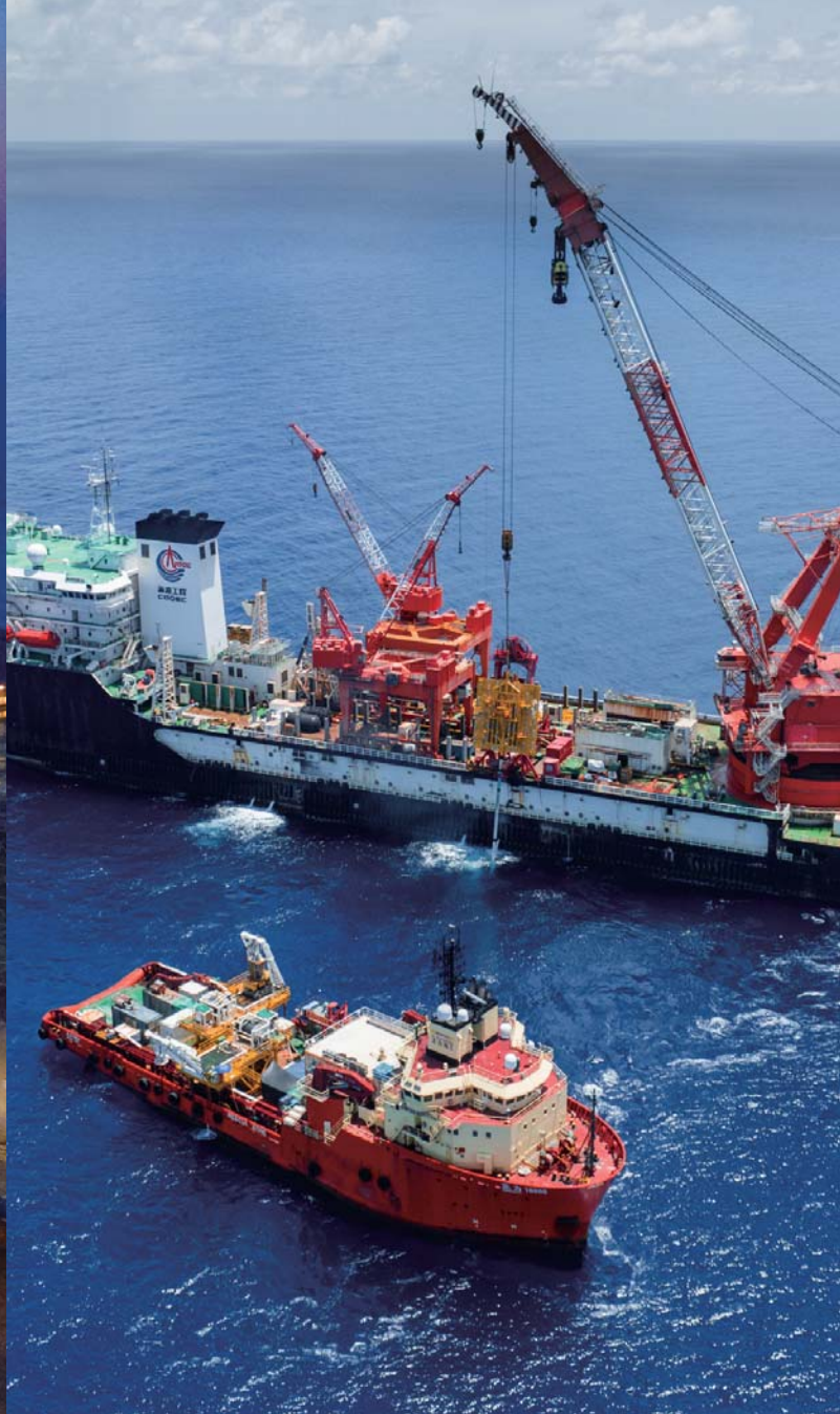
Submarine pipeline terminal installation site of "Shenhai-1" Phase-II Project
