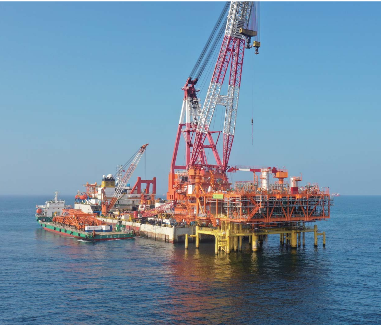
□ Offshore installation of WHPC block for Bozhong 19-6 Condensate Field Phase-I Project
