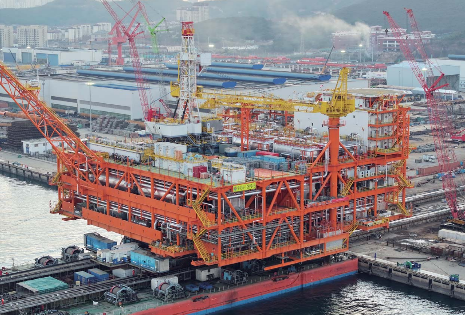
CEPQ platform slippage shipment of Suizhong 36-1 Secondary Adjustment Project
