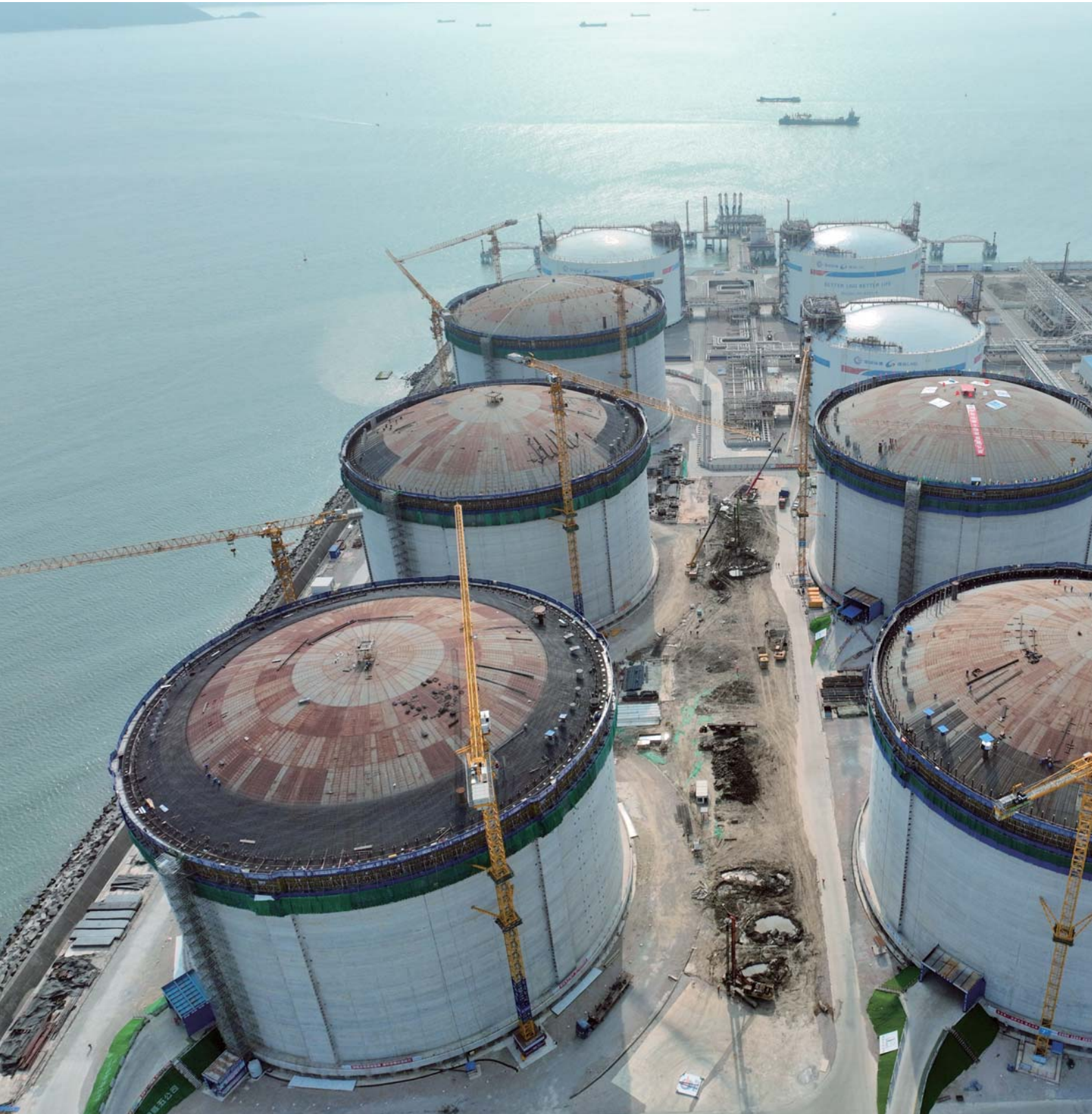
Construction site of Guangdong Zhuhai LNG Expansion Phase II Project
