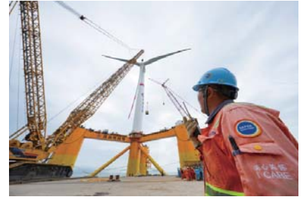
Final assembly site of "CNOOC Guanlan"
