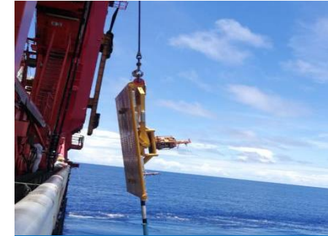
1,500m PLS Installation
