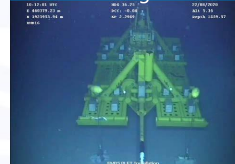
4.5in S-lay Folded PLET 1,500m depth
