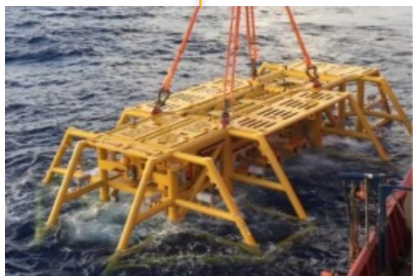
LH16-12 Manifold Installation 流花16-2 管汇安装
