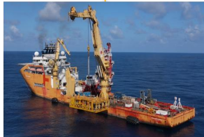
LS17-2 Manifold Installation 陵水17-2水下管汇安装
