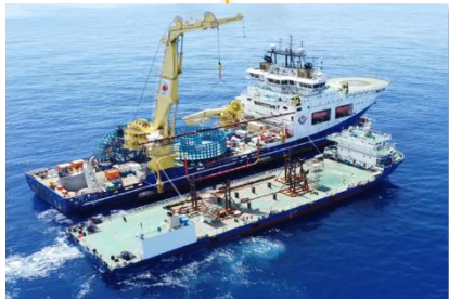
LH29-1 Jumper Installation 流花29-1 跨接管安装
