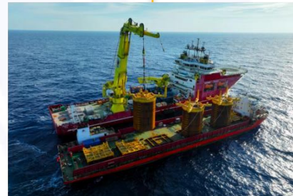
LS25-1 Suction Anchor Installation 陵水25-1二期吸力桩安装
