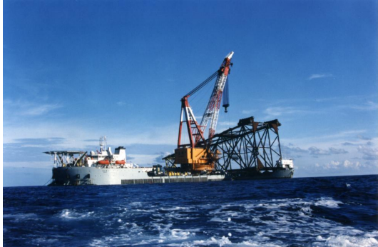
Lanjiang Derrick & Lay (3,800tons)
