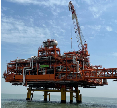
Ultra-high Pressure Gas Injection Platform
